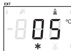
Fig. Frost protection is activated
